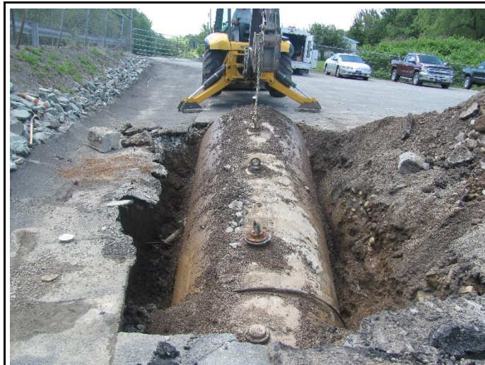
UST removal at the PennDOT Preston Center Stockpile, Wayne County, Pennsylvania
