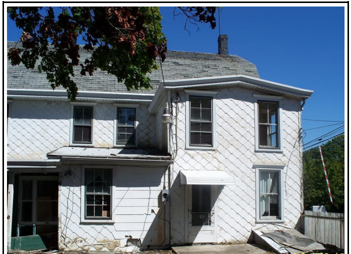
Asbestos abatement project in Hazleton, Luzerne County, Pennsylvania; PennDOT Engineering District 4-0
