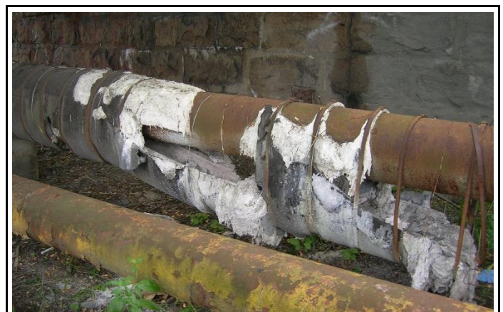
Asbestos abatement project in Franklin Borough, Cambria County; PennDOT Engineering District 9-0
