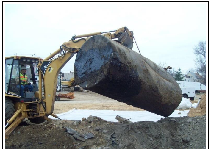
UST removal for the PennDOT I-95, Section CP2 Improvements Project
