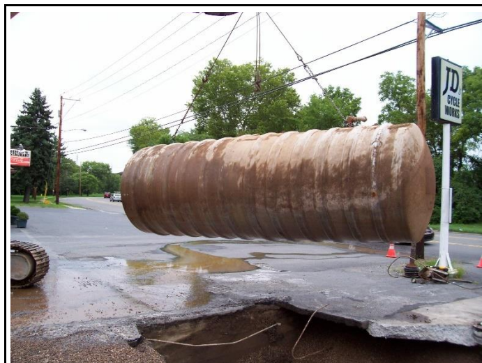
UST removal for the PennDOT S.R. 0412 Improvements Project, Bethlehem, Pennsylvania
