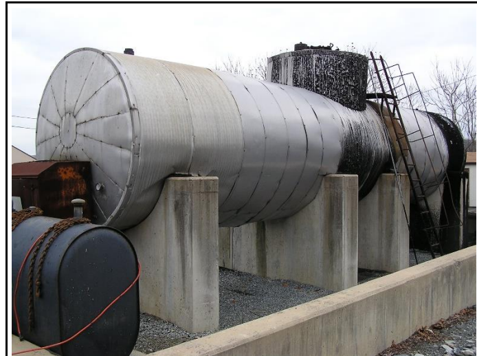
AST removal at the PennDOT Quarryville site
