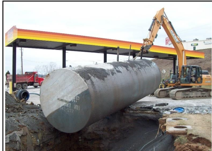
UST removal for the PennDOT I-83 Mt. Rose Avenue Improvements Project
