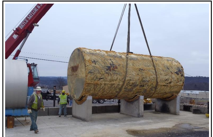
AST removal at the PennDOT Huntingdon Maintenance Facility
